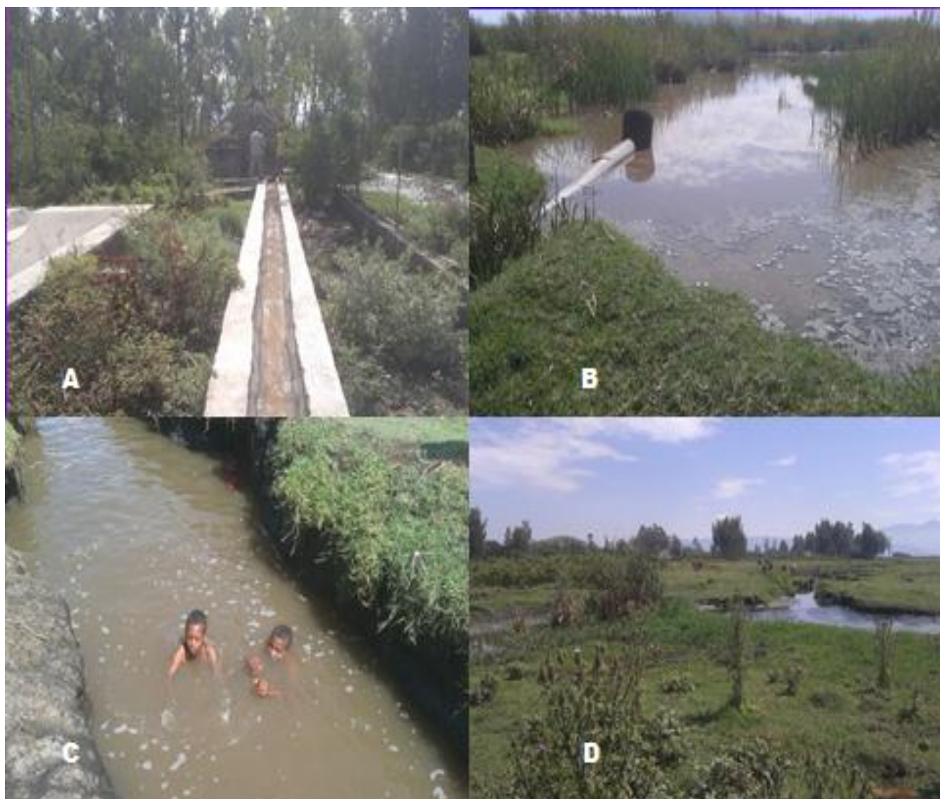
Fig.3.1. Concrete ditch (A) that takes the effluent from MHSDF into an open ditch that is directly discharged at the edge of the wetland (B) and flows down to the Boga stream. The effluent from BGIH-BF that flows to the edge of the wetland (C) confluent with the one from Moha and flows down to the Boeitch stream along the edge of the wetland (D). (Photo RT)
