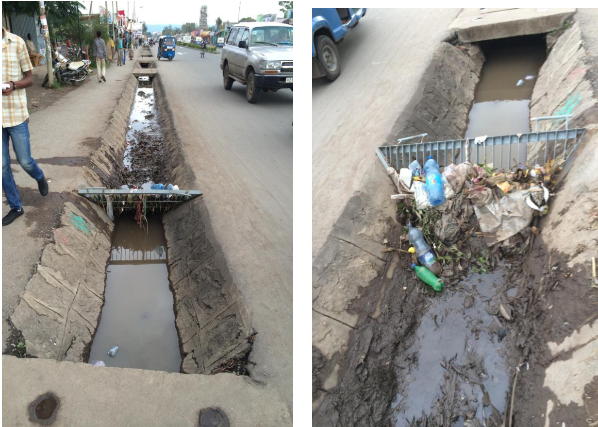
Fig. 3.4. Filtering racks (municipal waste trash trap) constructed along the drainage canal holds trash/solid wastes and helps to retain the trash and silt before reaching the hot inlet spots which also decreases the burden on storm water treatment ponds under construction along the lake shoreline by Hawassa Municipality (Photo by RT)
