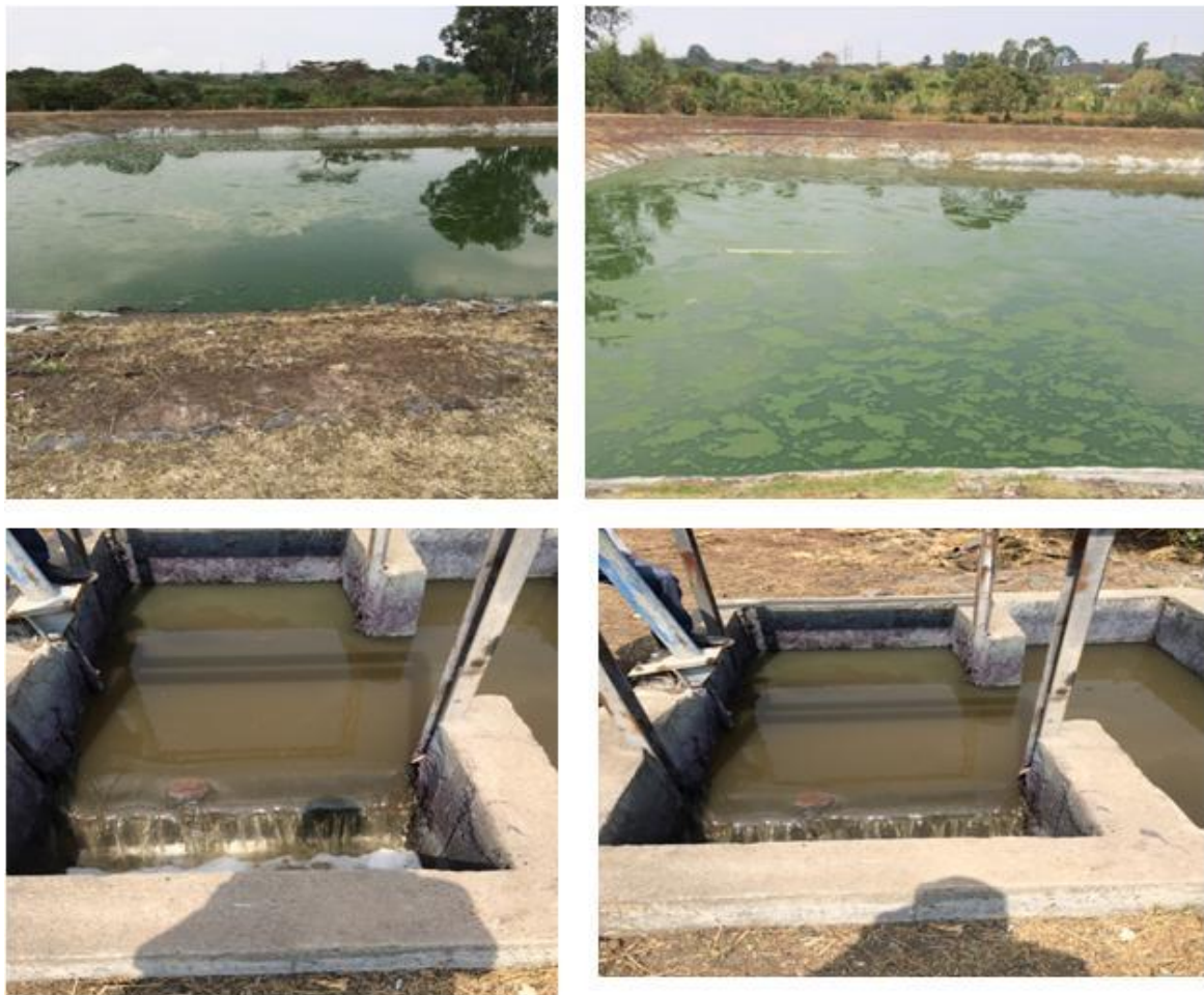
Fig 3.5. Biological lagoon outside the HTF: The effluent from the factory reaches the lagoon through underground channel by crossing the village. Note how damaged the ponds are. (Photo by RT)
